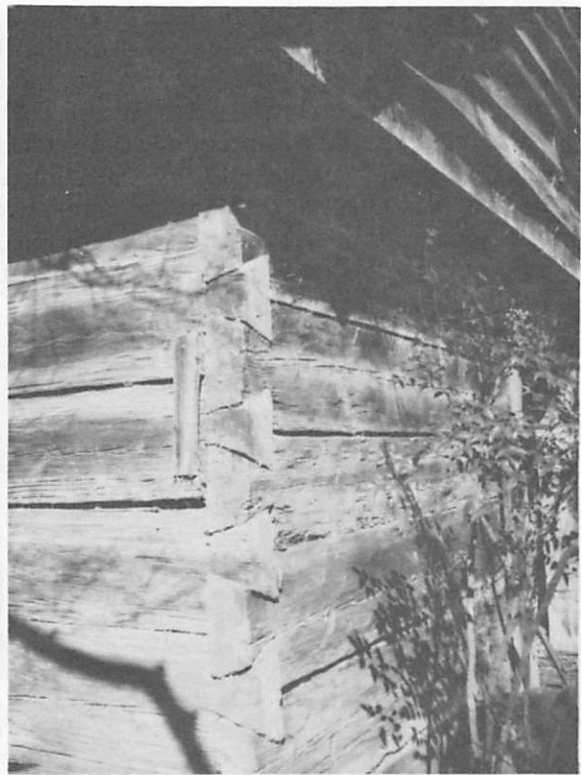
FIG. 15. An abundance of readily available timber provided building materials for almost every early structure in the region. Construction techniques varied. A Lexington County log structure (left) illustrates the German method of joining stripped logs with the saddle notch. Right, the English practice of dovetailing hewn logs is shown in a Richland County building.
