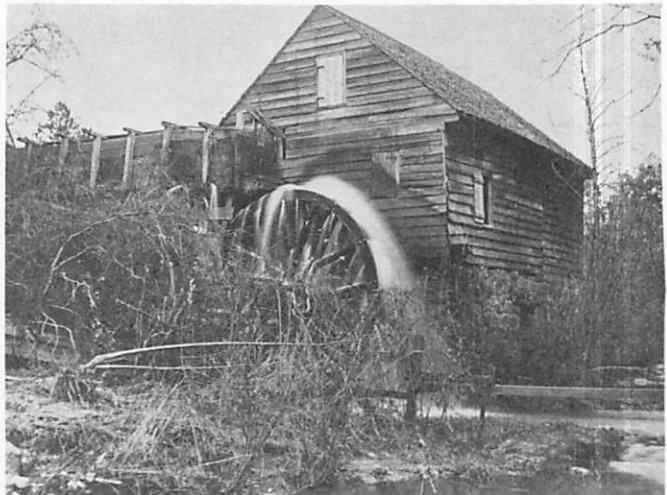
FIG. 16. Lumber and grist mills once dotted the region's numerous creeks and streams as the backcountry's principal early commercial enterprises. The above structure, with overshot wheel, was typical of hundreds of such mills, of which only scattered discarded millstones remain today.
