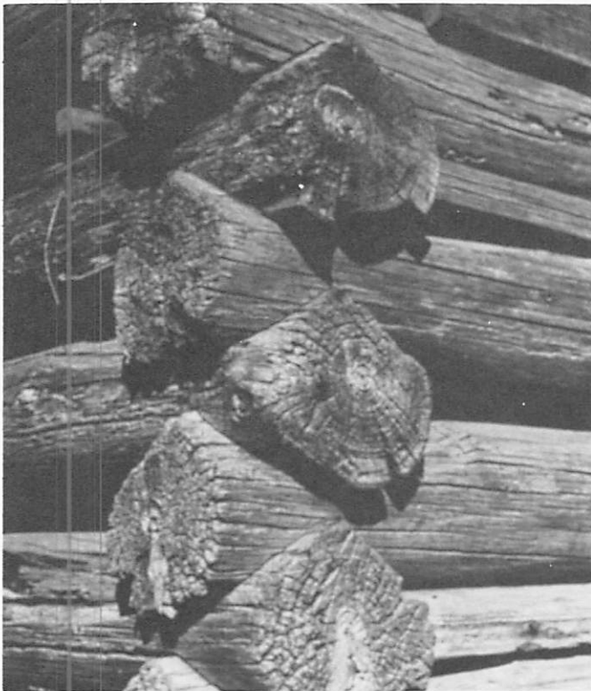
FIG. 15. An abundance of readily available timber provided building materials for almost every early structure in the region. Construction techniques varied. A Lexington County log structure (left) illustrates the German method of joining stripped logs with the saddle notch. Right, the English practice of dovetailing hewn logs is shown in a Richland County building.
